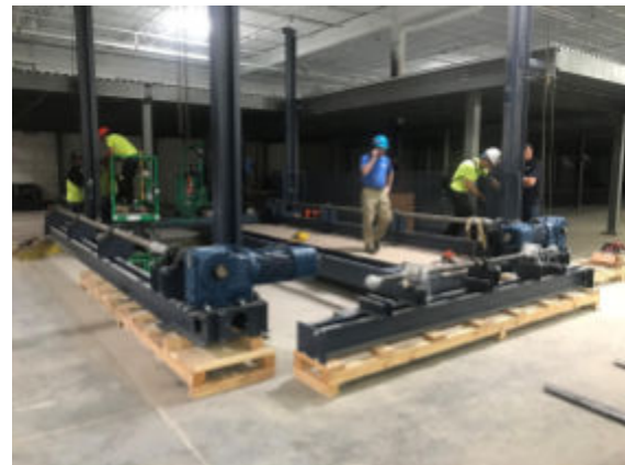
A controlled work zone helps separate installation activity from daily production and material handling traffic.
