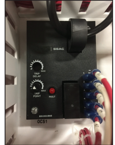
Overcurrent Sensor Figure 21-1
