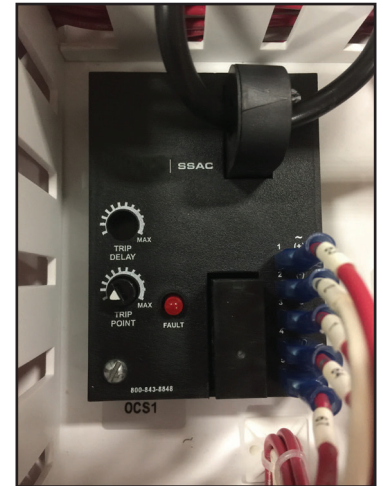
Overcurrent Sensor Figure 15-1
