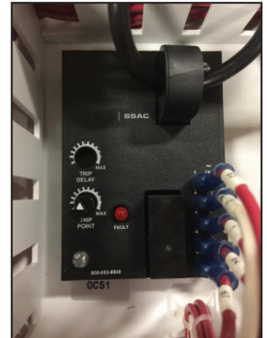
Overcurrent Sensor Figure 15-1
