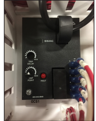
Overcurrent Sensor Figure 21-1
