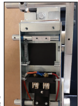
Single Contact PFlintlock Interlock Figure 17-22
