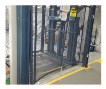
The alignment on conveyor systems can shift and create cart jams. Gates may need to be jiggled to make it open or close. Worn chains can lead to the rapid onset of wear on the teeth of the sprockets and loss of the teeth on the sprocket. Worn teeth on the lift sprocket becomes evident with an increase in noise, vibration, or choppy movement.
