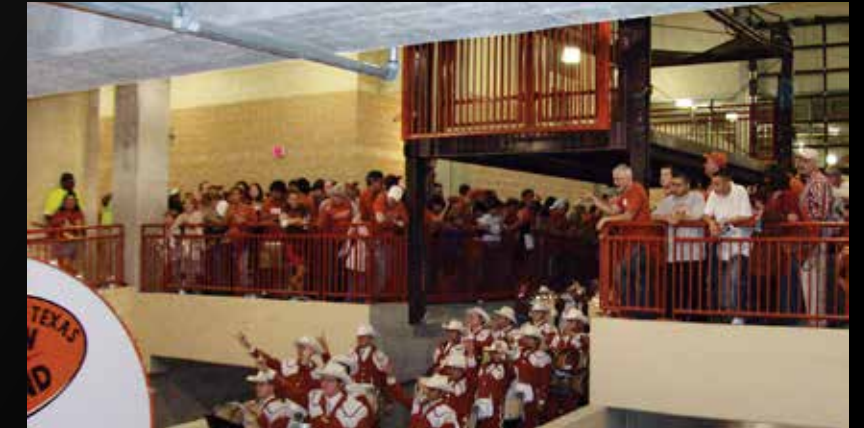
Stadium Concourse Lift – F Series Mechanical VRC 12' high clearance for the University of Texas Longhorns; 12,000 lbs. lifting capacity; fully ascends/descends in 30 seconds.
