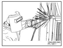
Weld Gate Header to Gate Posts Figure 16-77
