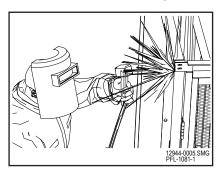
Weld Gate Header to Gate Posts Figure 16-27
